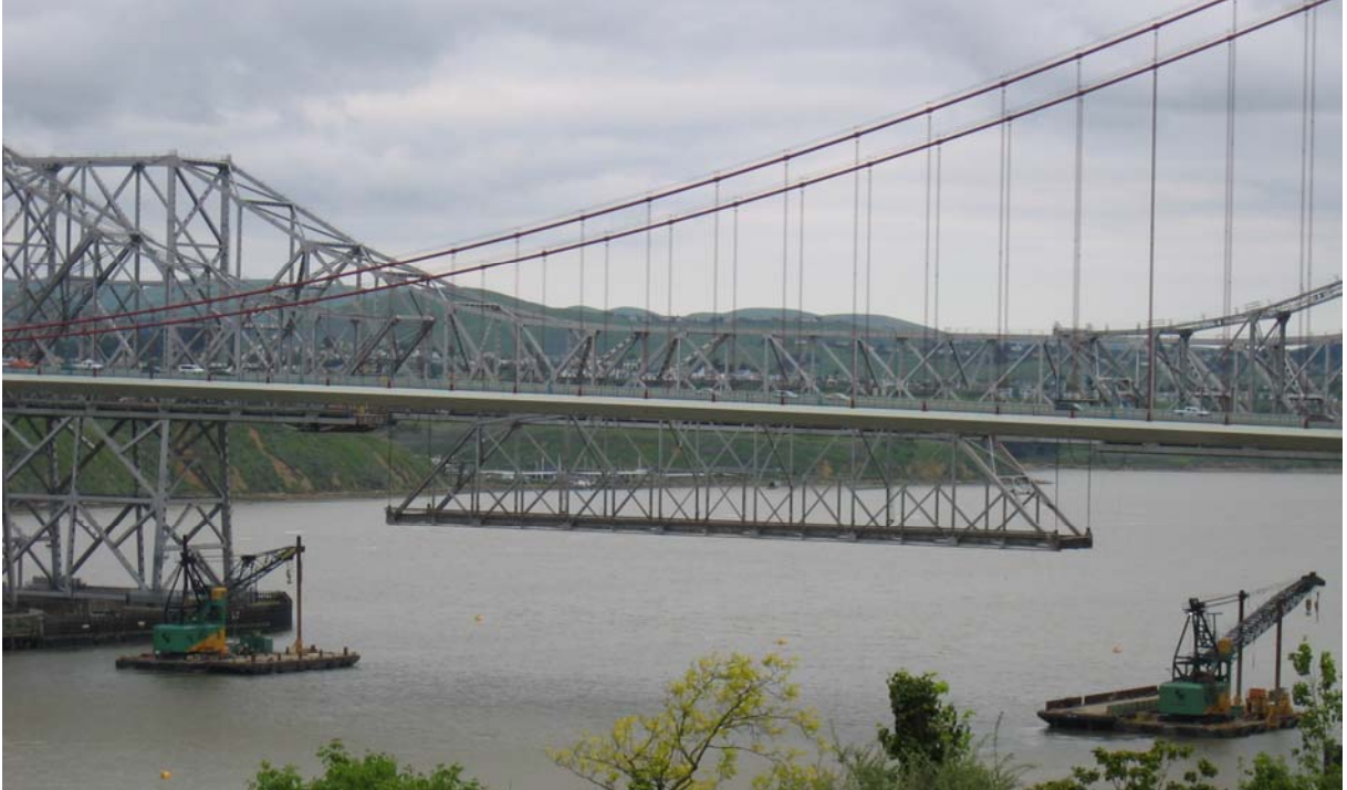
18" Increments. Carquinez Bridge Span Lowered for Off-Site Dismantling.
